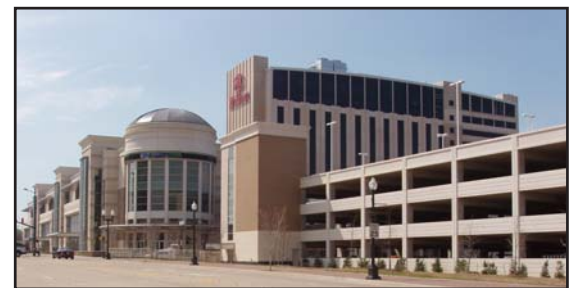
The completed Shreveport Convention Center.
