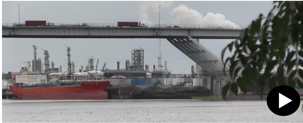
Ship Channel Bridge, Houston. (OIG video)
