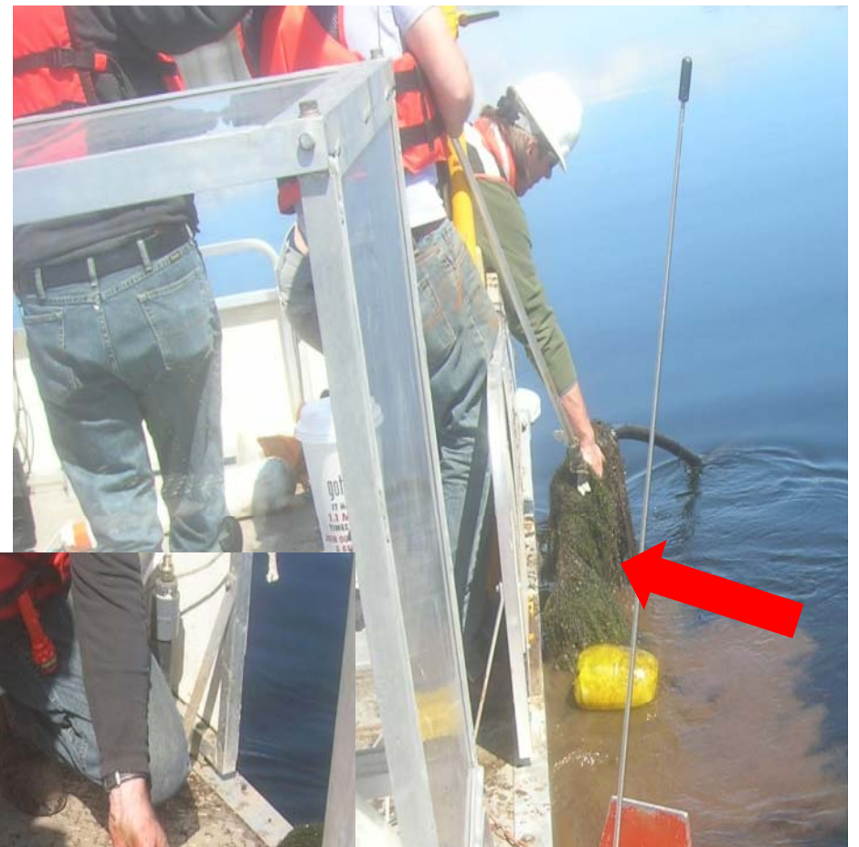
TID Intake Screen #4 being pulled to surface and covered with weeds and mud.
