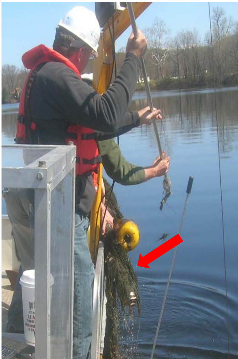
TID Intake Screen #3 being pulled from river and covered with weeds and mud
