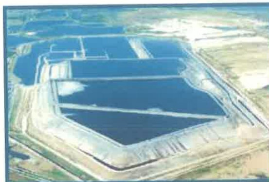
Figure B. Oblique view of a gypsum stack and Cooling water ponds.
