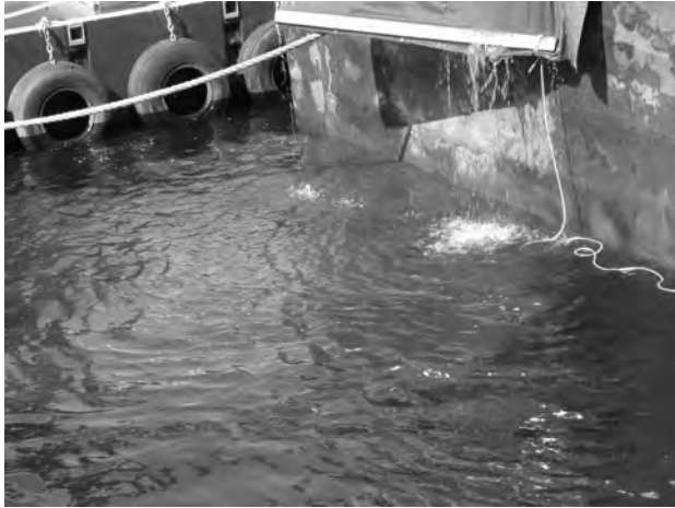
Figure 4. Dredge closure forces a slurry of sediment and water upward through the open top of the bucket, and leakage of incompletely closed buckets drops material onto the river surface. Hudson River dredging site, July 28, 2009.
