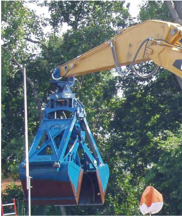
Figure 1. Hudson River dredge showing bucket suspended beneath superstructure.
