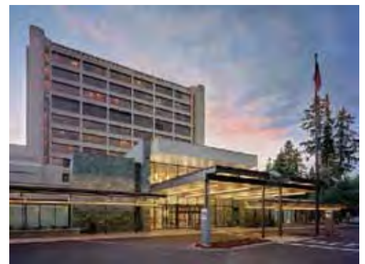
Providence St. Peter Hospital exterior
