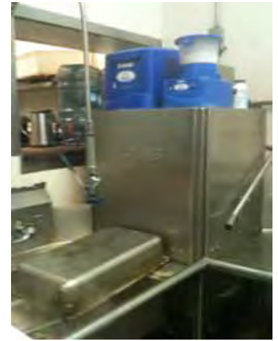
ENERGY STAR qualified dishwasher and high-efficiency pre-rinse spray valve installed at one of Uncommon Ground's locations
