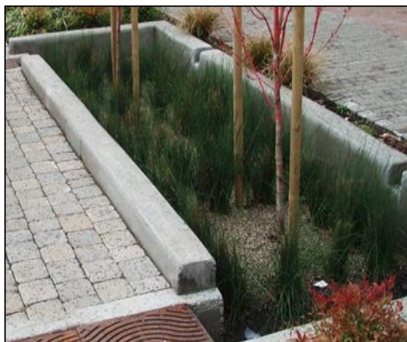
Figure 7 – Typical planter box (Source: Philadelphia Water Department, 2014)
