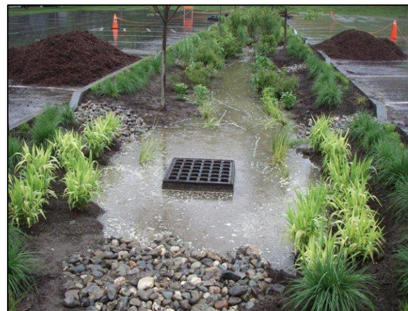
Figure 6 – Typical bioretention application (Source: Vermont Watershed Management Division, 2013)
