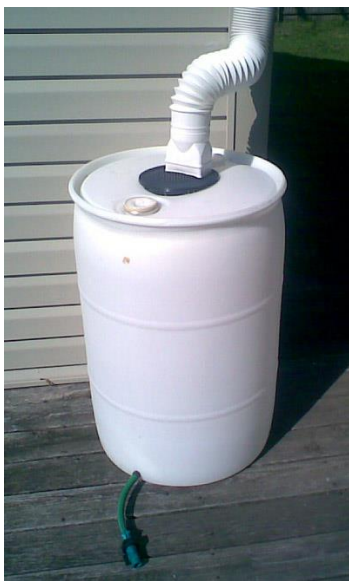
Figure 5 – Typical Rainwater harvesting tank in an urban setting (top) (Source: www.sswm.info ) and typical rain barrel application (bottom) (Source: www.rainbarrel.org )
