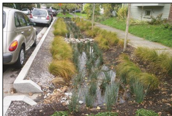
Figure 8 – Typical urban bioswale (Source: American Forests, 2012)
