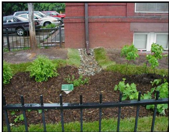
Figure 4 – Typical downspout disconnection configuration (Source: LID Center, 2005)
