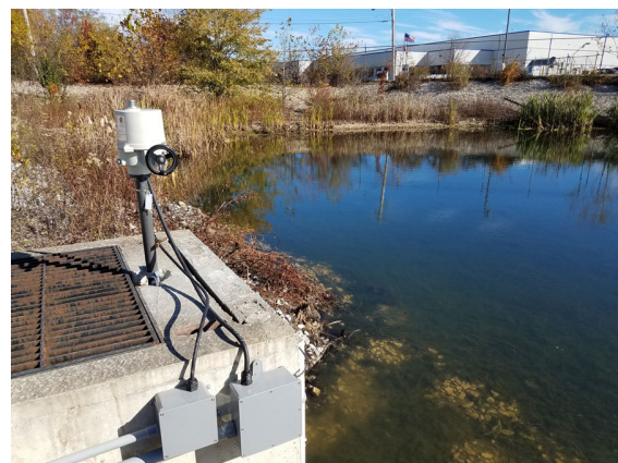
Figure 1. CMAC installation on the existing outlet control structure.
