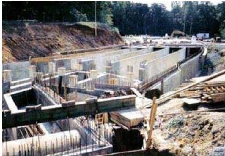
Figure 1. The 2.7 MG Canby Park CSO Storage Basin under construction.
